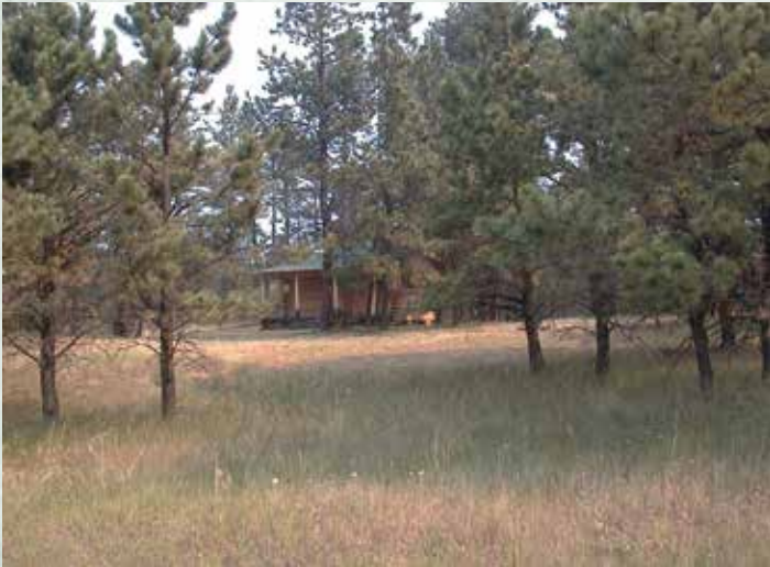
This cabin appears at first glance to not have any problems but look closely at how thick and dense the forest is, how tall the brown grass is, and the firewood pile under and near the deck. See the photo to the right after the wildfire arrived.
