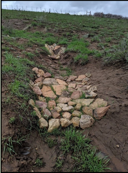
Rock rundown with vegetation growing between cracks. Photo: Kristina Kline, Bird Conservancy of the Rockies
