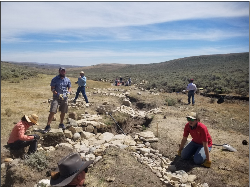
August 2021 Workshop— Series of Rock rundowns and One Rock Dams along the drainage
